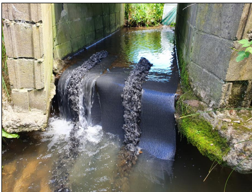
Figure 6. Two flexible rubber ramps with mussel-rope at the culvert outlet.
