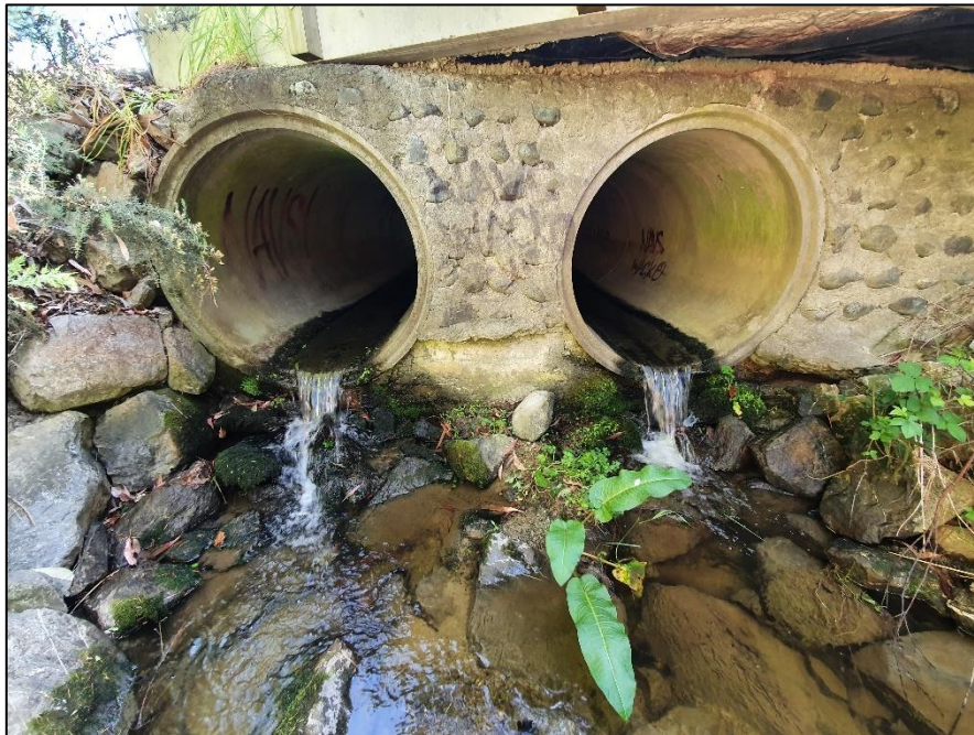
Figure 2. Perched culverts at William's Creek prior to remediation.
