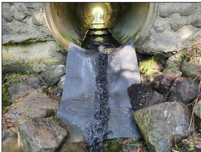
Figure 8. Flexible rubber ramp with mussel-rope
