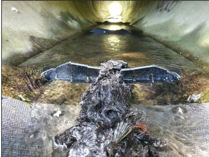
Figure 7. V-baffle and mussel-rope at the culvert outlet.
