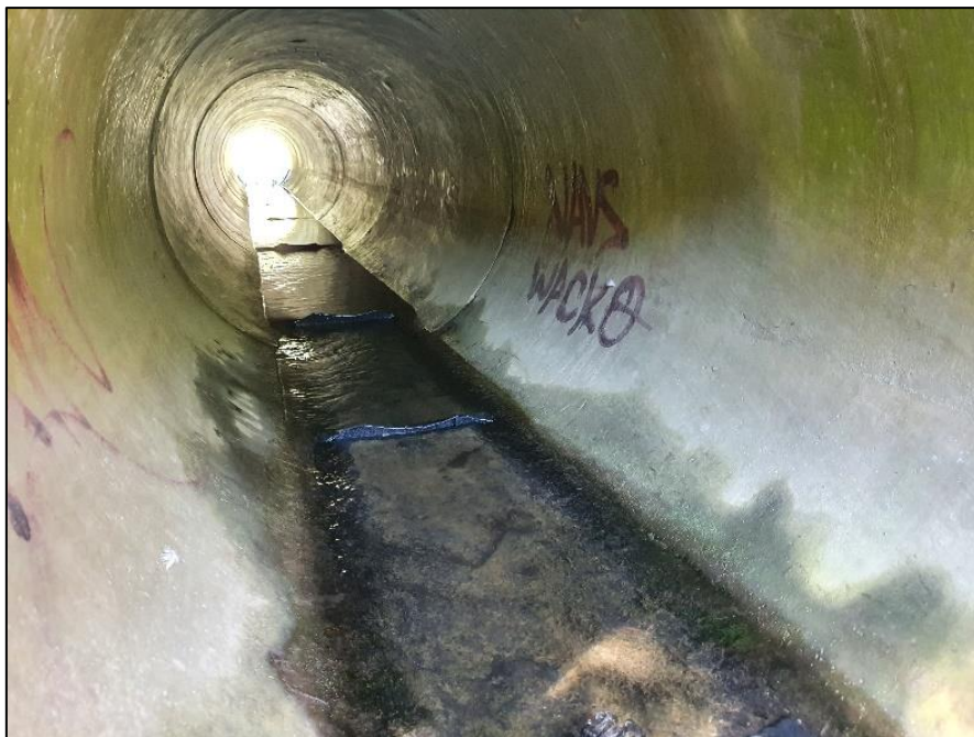
Figure 6. Flexible baffles within the true left-hand culvert pipe.
