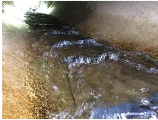
Figure 1: Flexible baffles placed on the invert of a curved culvert (left), 450mm wide flexible baffles within the 9.3% grade section of the Todd Valley Stream Culvert (right).
