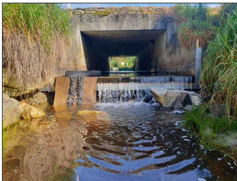
Figure 2. Dominion Stream culvert remediated with a flexible rubber ramp.
