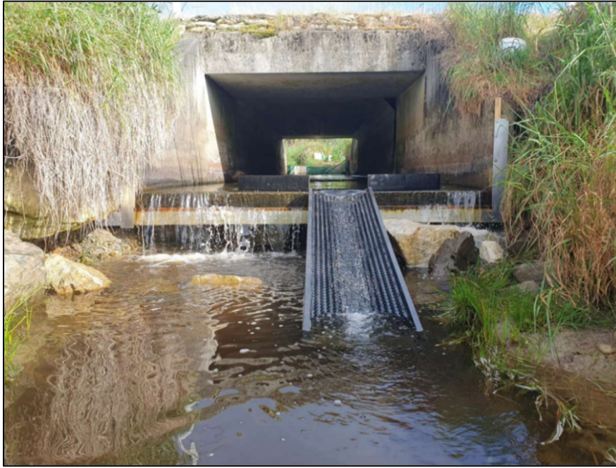
Figure 3. Dominion Stream culvert remediated with a single floating fish ramp.
