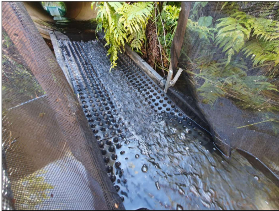
Figure 15. Remediation at Williams Creek showing a floating ramp.
