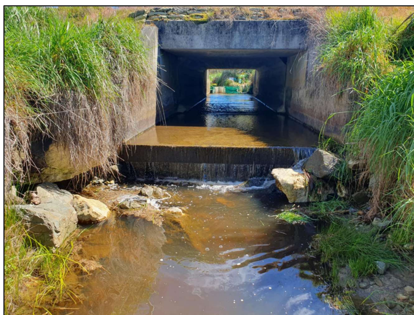
Figure 1. Perched box culvert at Dominion Stream prior to the beginning of the fish passage evaluations, October 2024
