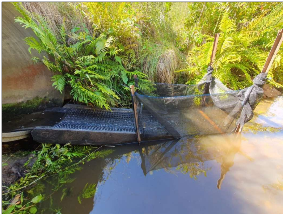
Figure 17. Single floating ramp and outlet net at the Williams Creek round culverts.
