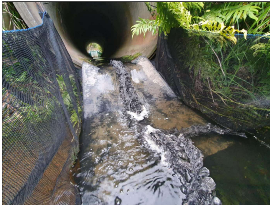
Figure 14. Remediation at Williams Creek showing a flexible rubber ramp.
