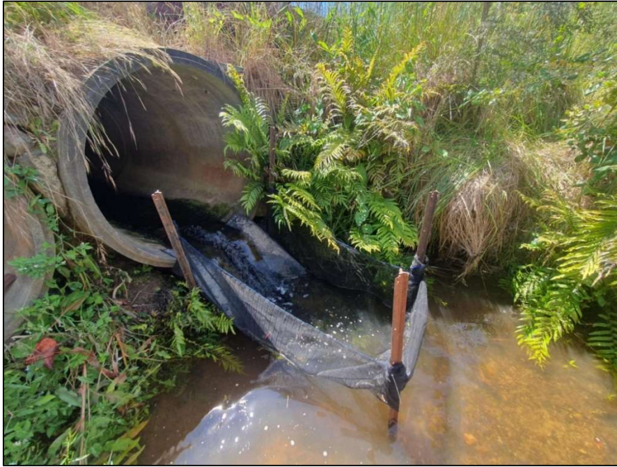
Figure 18. Flexible rubber ramp and outlet net at the Williams Creek round culverts.
