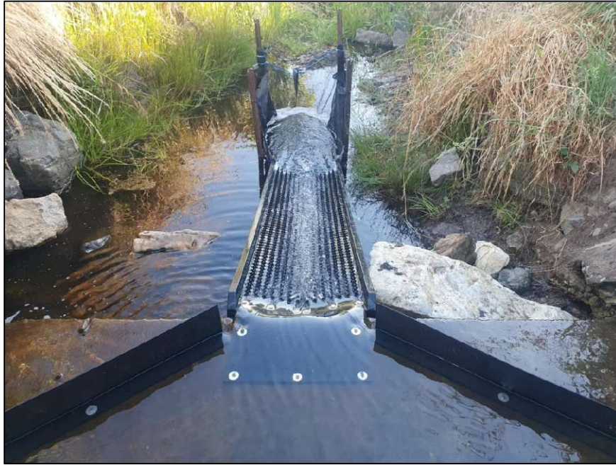
Figure 10. Single floating ramp and outlet net at the Dominion Stream box culvert.
