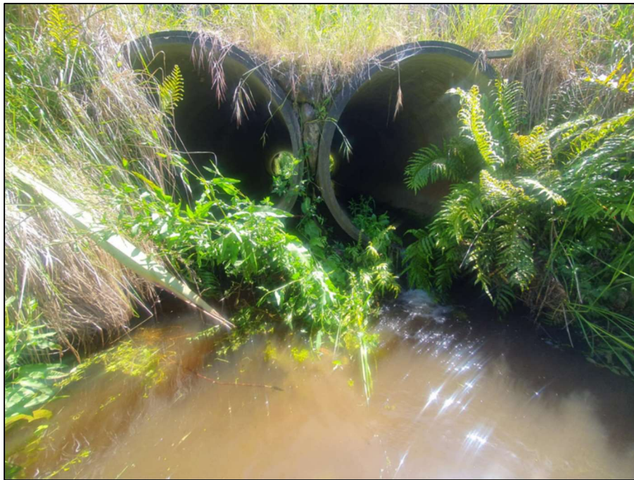
Figure 13. Perched round culverts at Williams Creek prior to the beginning of the fish passage evaluations, November 2024
