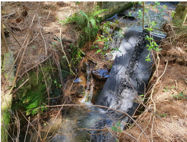
← Culvert apron fitted with a flexible ramp, mussel-rope and flexible baffles.
