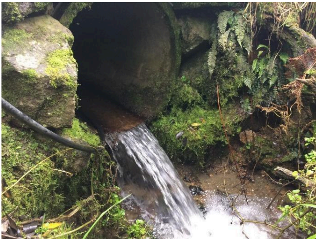
Perched culvert pipe
